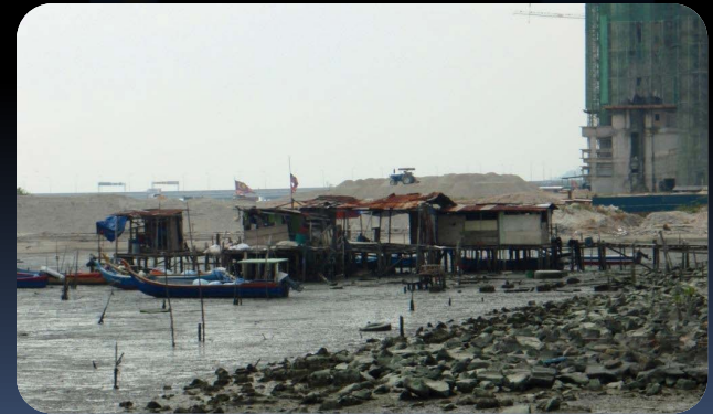
Land reclamation, fishing village Penang
